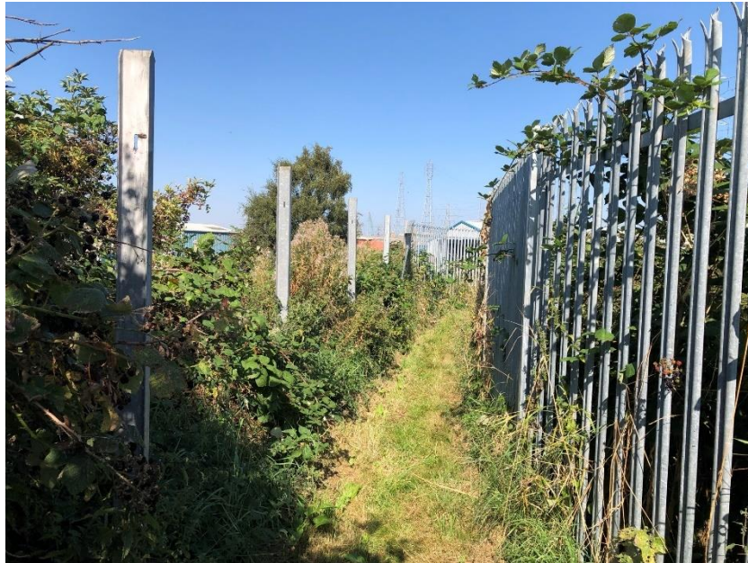
Figure 1-7 Broken sections of fencing and general sense of neglect along the path.
